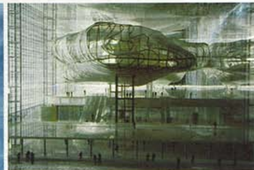
MASSIMILIANO FUKSAS'S CONGRESS CENTER (LEFT AND ABOVE) IN ROME, OPENING IN EARLY 2008, CONTAINS A STEEL-AND-TEFLON "CLOUD" — THE IDEA FOR WHICH CAME TO FUKSAS ONE DAY WHEN CLOUDS WERE BLOWING IN A STRONG WIND.
