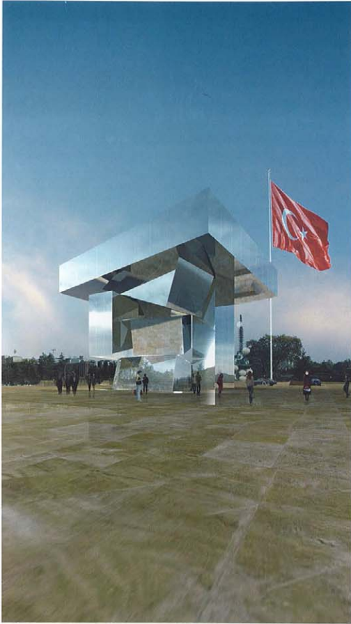
Vakko Headquarters and Power Media Center, Istanbul, Turkey, 2007-9. Vakko, Turkey's preeminent fashion house, and its sister company, Power, commissioned REX to design their new headquarters using a preexisting, four-story concrete skeleton. The outer ring is clad in a thin sheath of self-supporting slumped glass panels that render traditional window frames unnecessary. Embraced by the ring is a cluster of steel volumes that house Vakko's large program of unconventional spaces, including offices, showrooms, conference rooms, an auditorium, television studios, radio production facilities, screening rooms, and a museum.
