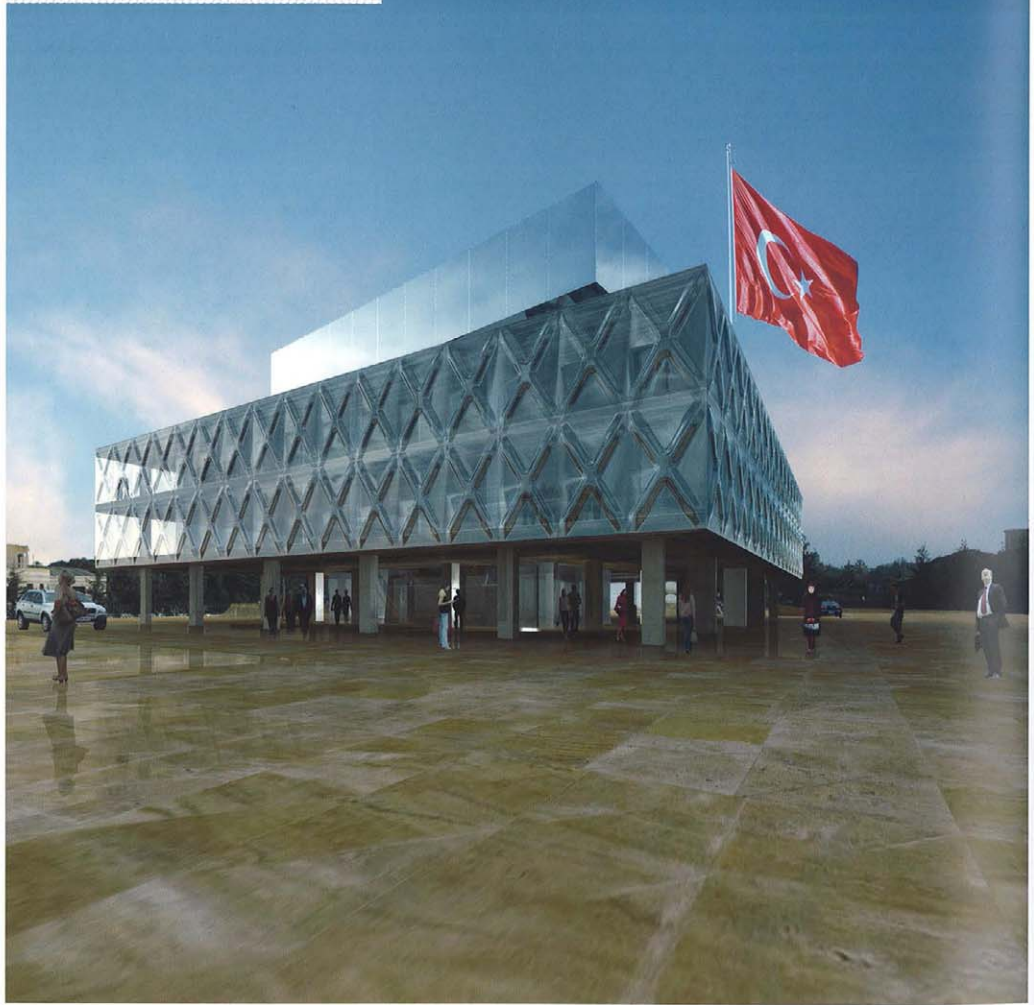
Vakko Headquarters and Power Media Center, Istanbul, Turkey, 2007-9. Vakko, Turkey's preeminent fashion house, and its sister company, Power, commissioned REX to design their new headquarters using a preexisting, four-story concrete skeleton. The outer ring is clad in a thin sheath of self-supporting slumped glass panels that render traditional window frames unnecessary. Embraced by the ring is a cluster of steel volumes that house Vakko's large program of unconventional spaces, including offices, showrooms, conference rooms, an auditorium, television studios, radio production facilities, screening rooms, and a museum.
